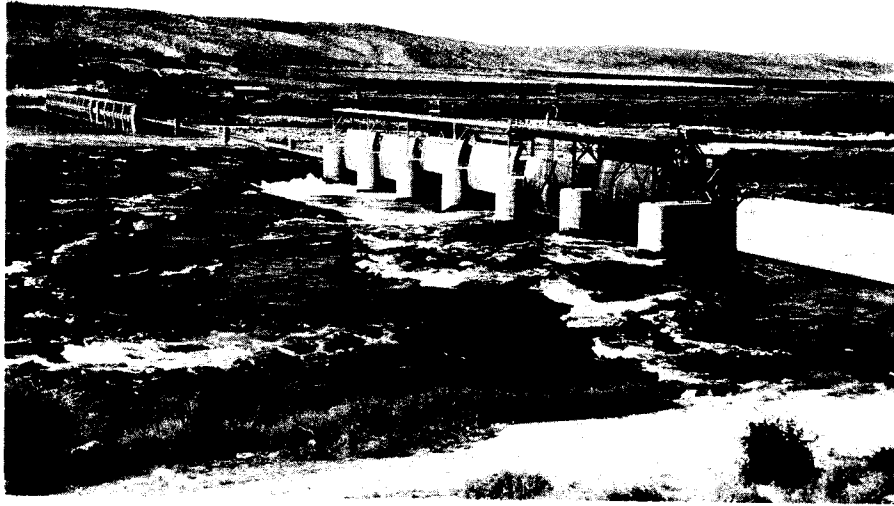
Plate 5. Diversion dam at Upper Salmon Falls. (Idaho Power Company photograph)
