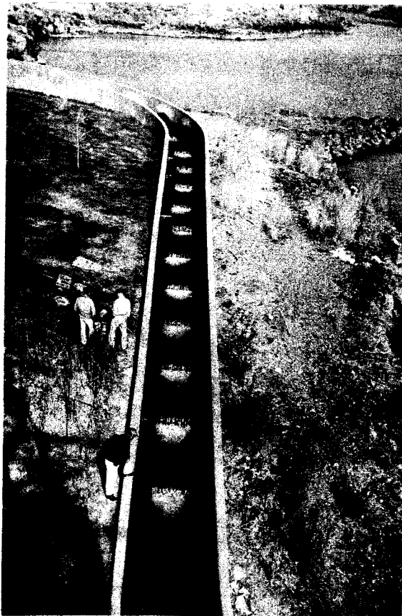
Plate 35. Reduced water flow in fishway over Lower Salmon Falls Dam in preparation for the collection of fish from pools with electrical shocker equipment.
